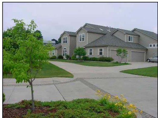
New areas of high-density housing options have recently been developed in Orrville.
