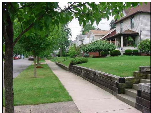
Orrville's traditional neighborhoods are characterized by grid streets and houses on smaller lots.
